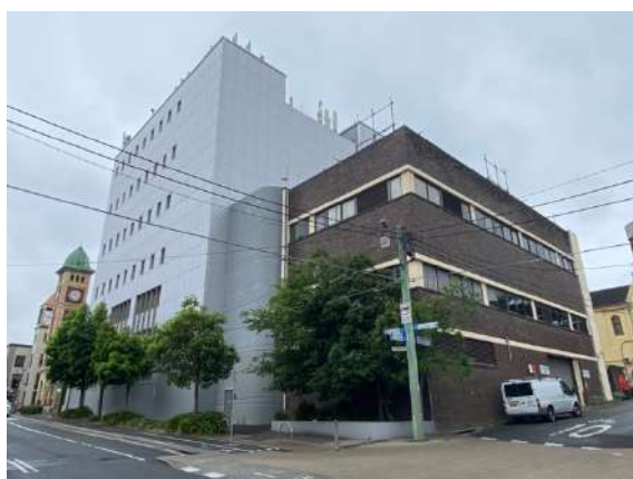
Figure 4: Photo taken from the corner of George and Turner Street showing the 1957 telephone exchange building on the left and the 1974 building on the right.
