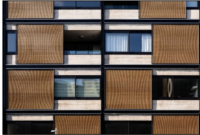
Figure 2: example for screens on an apartment building
