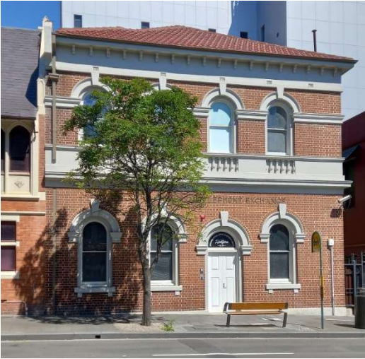
Figure 3. 117A Redfern Street, Redfern. Source: https://www.facebook.com
